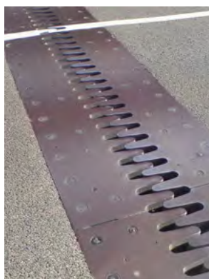
The expansion joint in a bridge.
